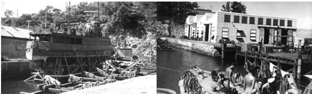
Left: HMAS Watcher in the Basilisk Slipway. Right: The naval repair workshop at Basilisk.
