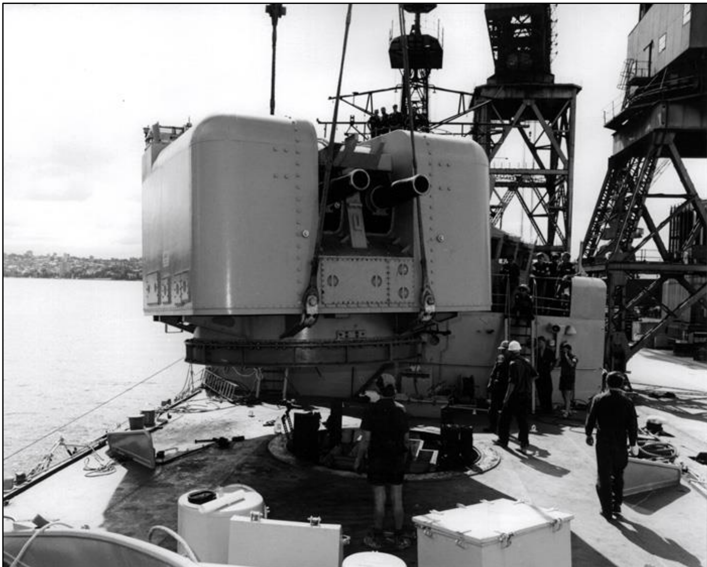
4.5inch gun turret being mounted on HMAS Yarra at Garden Island. c1970s
