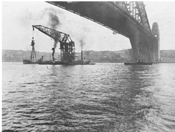
The floating crane Titan, being towed under the Sydney Harbour Bridge with the foremast of HMAS Sydney in 1929. The mast is to be installed at Bradleys Head.
