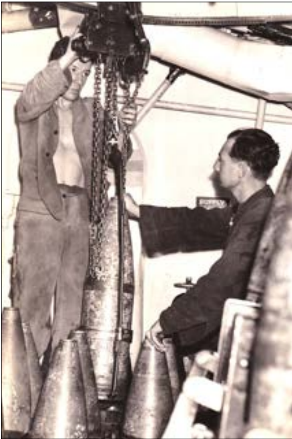
Above: Shell-room, HMAS Australia, in February 1943.
