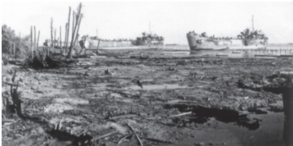
Tarakan: LST's sitting high and dry on the muddy beachhead at Tarakan waiting for the tide to float them off. These muddy beaches were a problem to engineers unloading stores.
