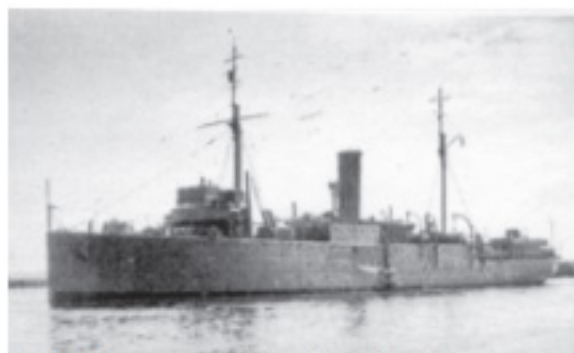
HMAS PLATYPUS - 1946, final operational appearance. Topgallant masts struck; gun mounted aft.
