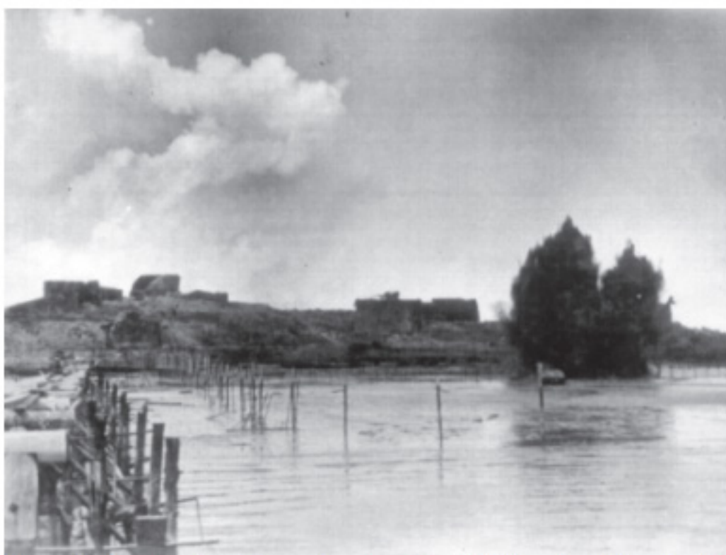
Up goes the wire - Australian engineers, going ashore ahead of the infantry in the Tarakan landing, successfully blew up wire defences in the shallows. ( Official photo MH 90909 )
