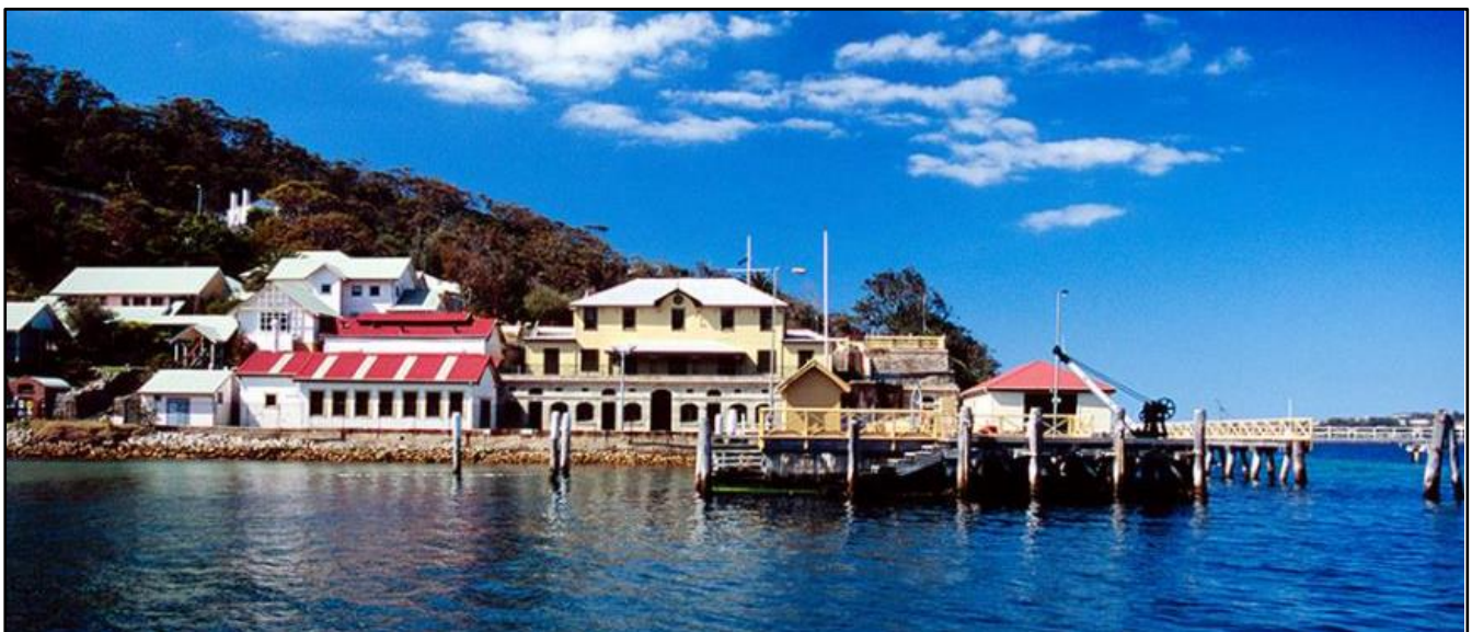
Submarine Mining Corps buildings at Chowder Bay as preserved today.
