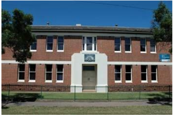
Naval HQ SA – Keswick Barracks South Australia
