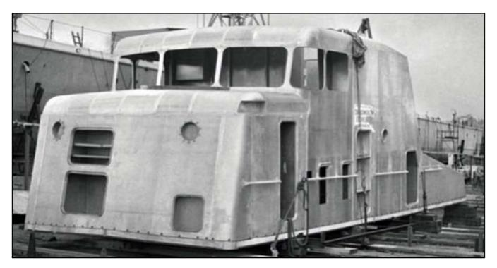
During construction of the first boat, HMAS *Attack*, in Brisbane, the weight of every piece of equipment taken on board and any removed was recorded. The person given this task took his
